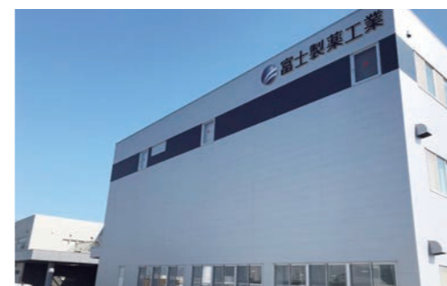
Management and welfare building completed in August 2020
