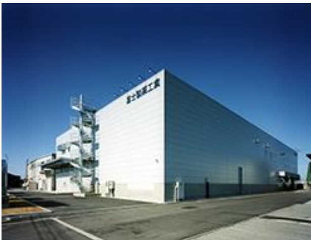
Injectable manufacturing plant (Fuji)
