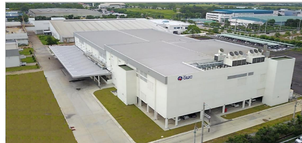
Injectable manufacturing plant (OLIC)
