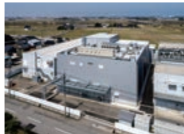
Newly constructed sixth drug production building
